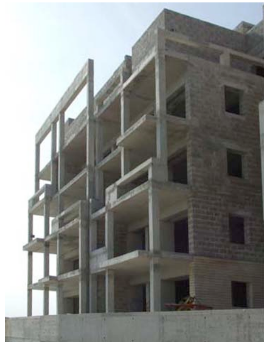
Fig 10. The seaward concrete screen during construction
