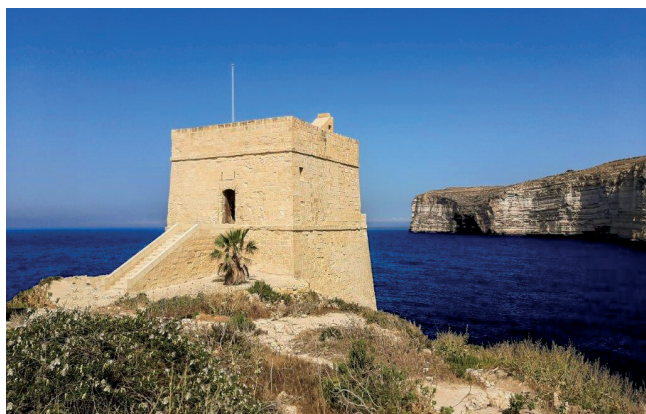
Xlendi Tower built by the Knights [Photo: Giovanni Zammit].
