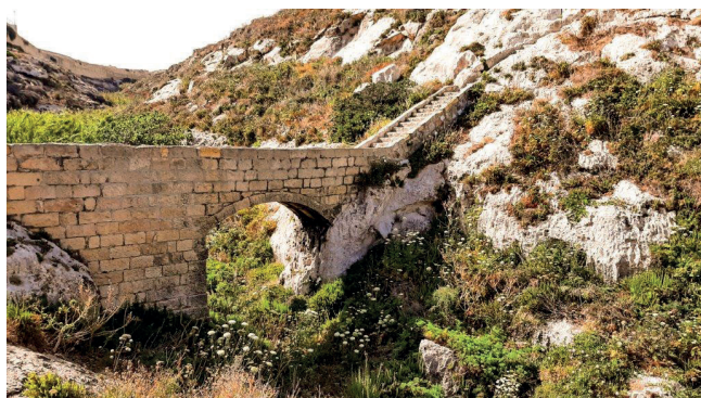
The bridge over the inlet Il-Kantra [Photo: Giovanni Zammit].
