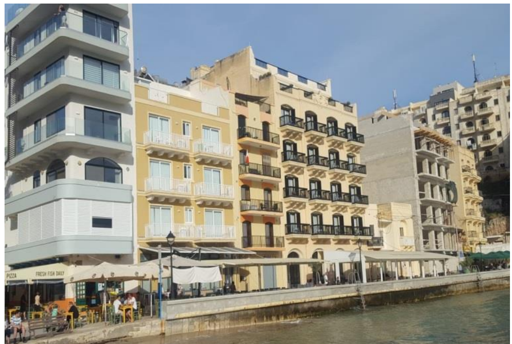
Figure 5. Businesses located along the promenade of Xlendi Bay.
