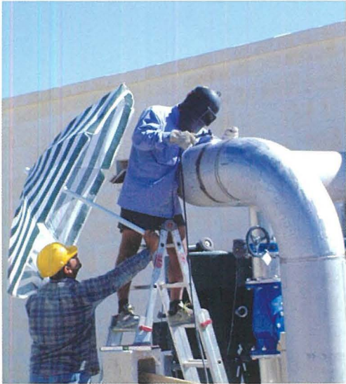
During construction works.
