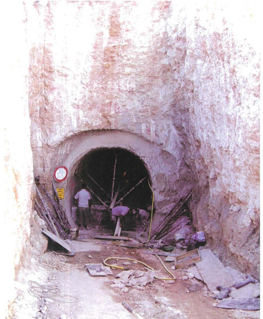
North sewage infrastructure gallery works-in-progress.
