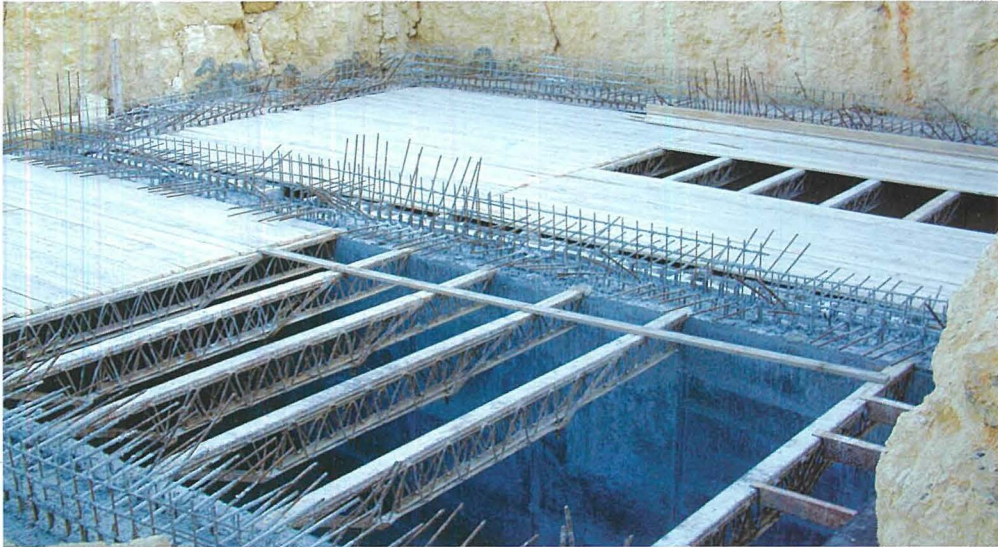
The San Blas pumping station under construction.
