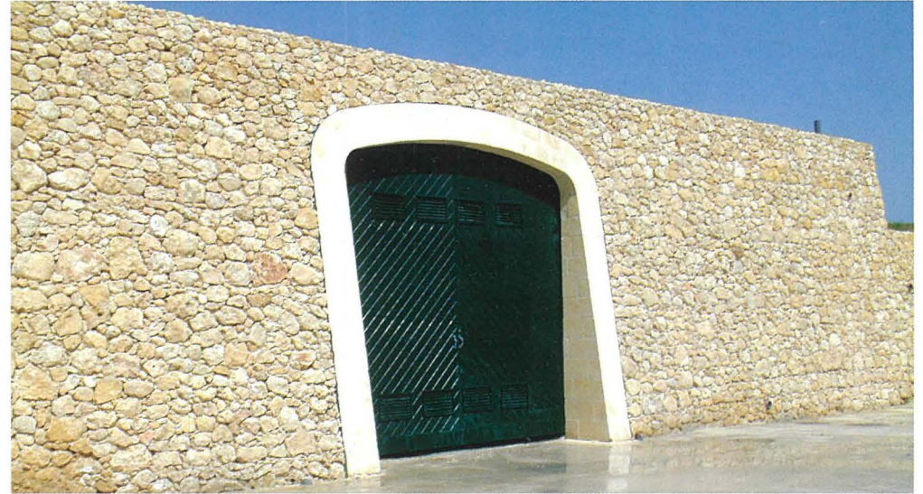
The Gharb pumping station.
