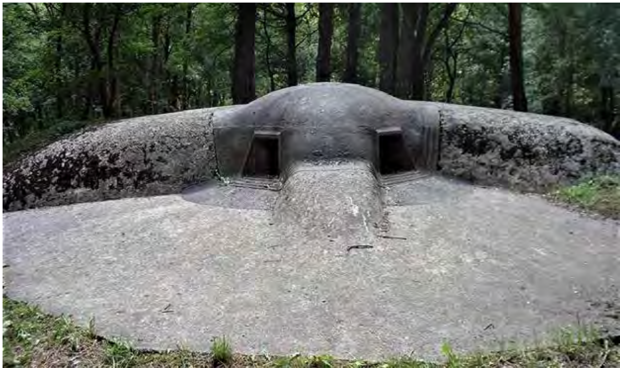
Abb. 07: Standardisierter MG-Kampfraum des Typs Casemate Pamart im Vorfeld des Forts Souville, Source: wikipedia to Commons by Bloody-libu using CommonsHelper. Author. The original uploader was Clicgauche at French Wikipedia.
