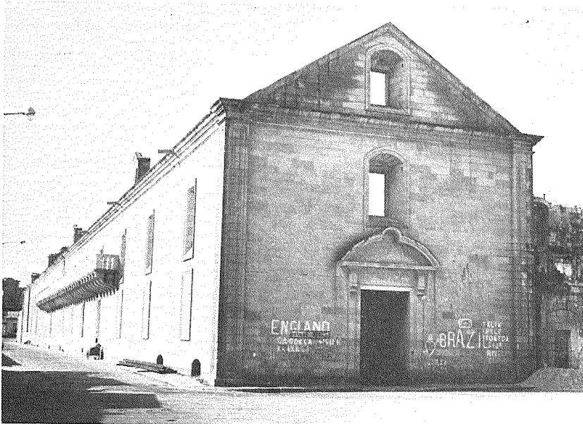
15. The shell of the Sacra Infermeria before restoration.
