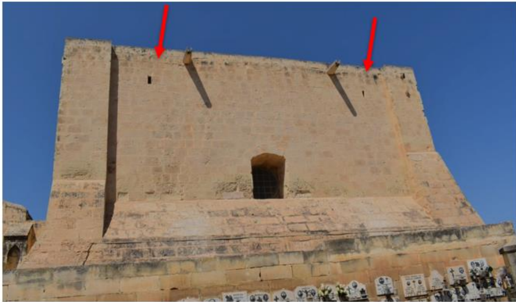
Figure 9. South side of the Chapel of San Girgor. Arrows indicate lookout windows. Photograph by author, October 2020.
