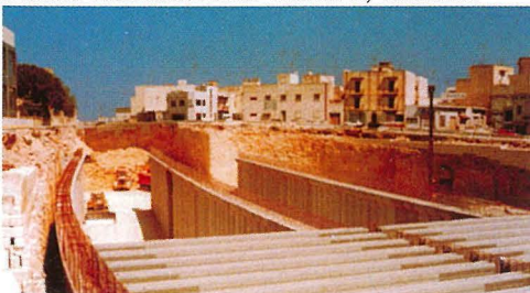
Msida multi-level intersection
