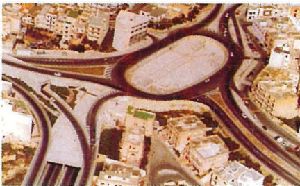
Msida multi-level intersection
