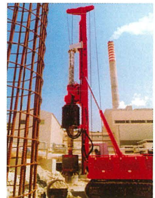
Piling works for Enemalta, gas turbine foundations
