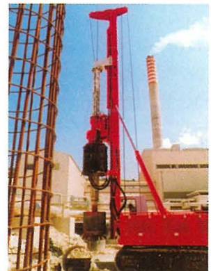
Piling works for Enemalta, gas turbine foundations
