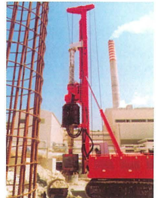
Piling works for Enemalta, gas turbine foundations
