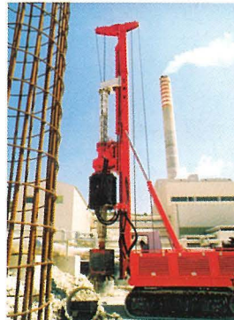
Piling works for Enemalta, gas turbine foundations
