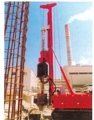
Piling works for Enemalta, gas turbine foundations
