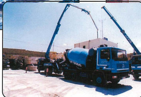
RMC and Concrete Pump
