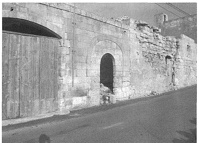
The last lime kiln that operated in Munxar.
