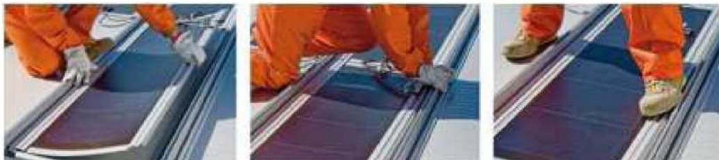
Figure 12: Thin Film clip on systems
