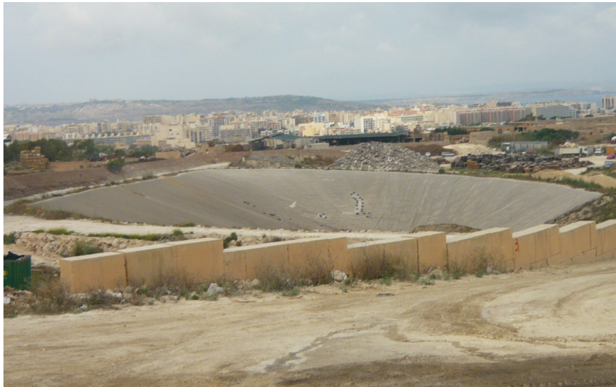
Figure 10: The new Ghallis Landfill under construction
