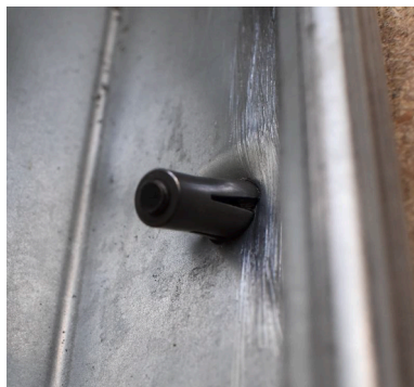
Fig. 14. Failure of specimen 1-P15-P3 – locking nut bearing into the steel sheet.
