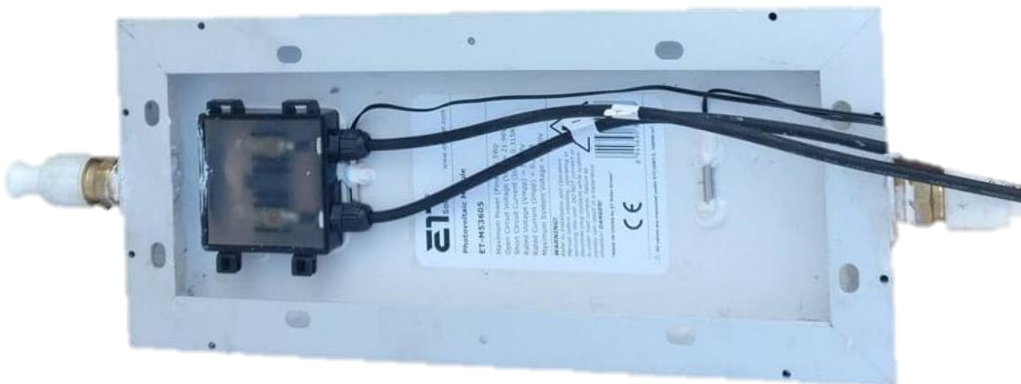
Figure 56: Junction box electrically insulated with resin, and Hep 2 O fittings installed.
