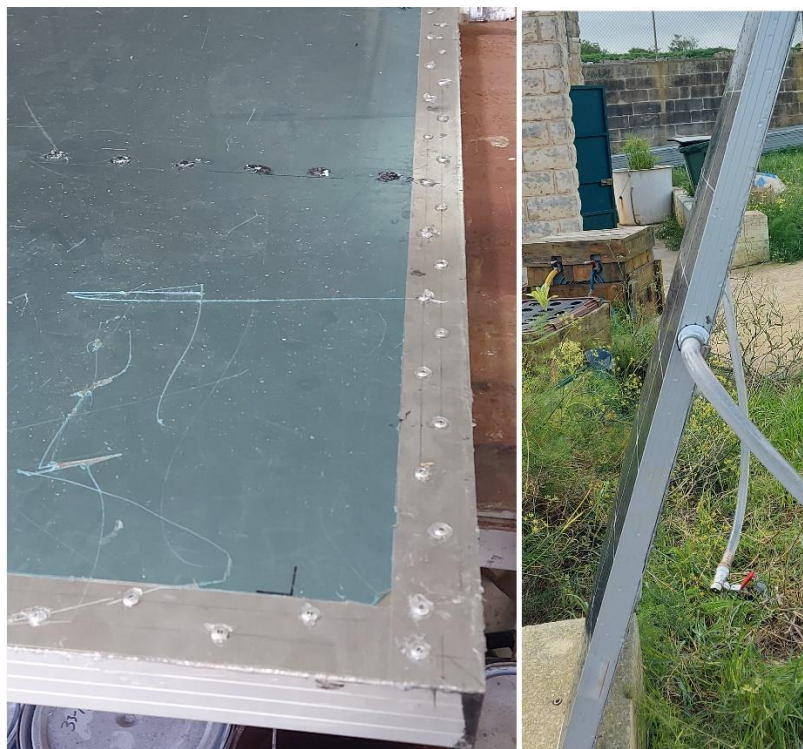
Figure 76: Aluminium sheet attached to the back of PV panel (Left) and filled PV panel at a high inclination angle showing bending of glass (Right).
