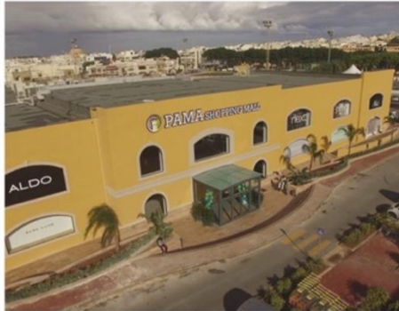
2: indoor shopping mall (Pama, Mosta)
