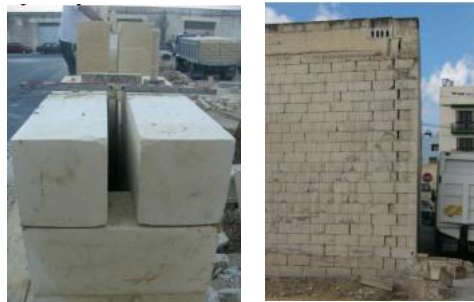
Figure 28 (left) Two skins of 230mm soft stone with a 50mm cavity, total 510mm and (right) Two skins of 160mm soft stone, typically with no cavity, total 360mm Source: (Buhagiar & Tonna, 2012)
