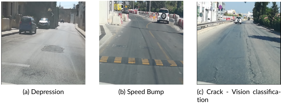
Figure 4.15: Field Testing Results: Visual Examples of Speed Bump, Depression, and Crack Anomalies
