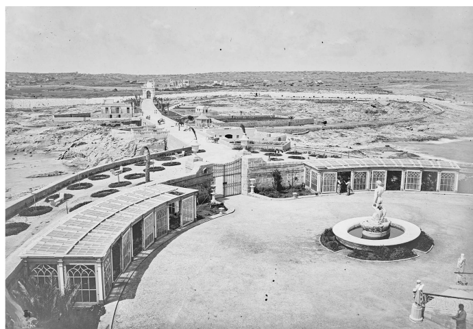
Figure 8. Photograph by Richard Ellis showing the access gate (top left) in the wall that enclosed the Dragonara Palace and the surrounding garigue grazing land. Late 19th century (reproduced by courtesy of the Richard Ellis Archive—Malta. M52-02).
