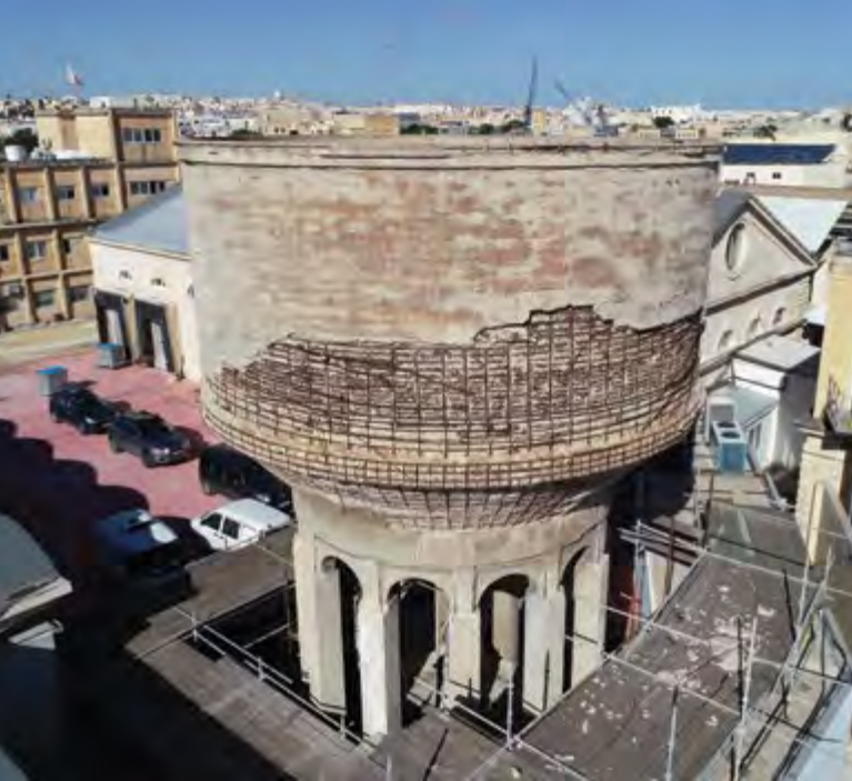
The tower before and after restoration.
