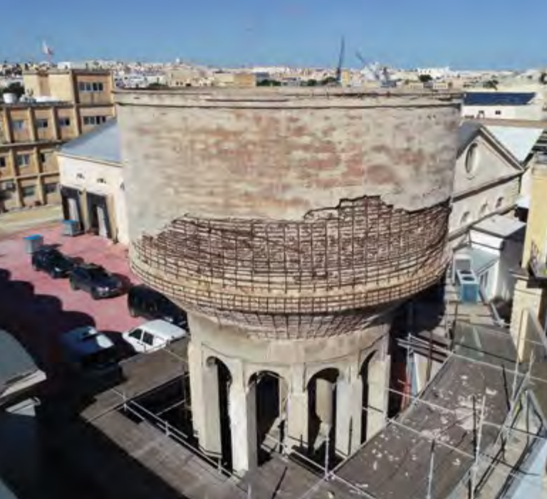
The tower before and after restoration.
