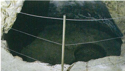
A sheared conical well that clearly shows the shape of these water storage vessels, typically found across the Maltese Islands
