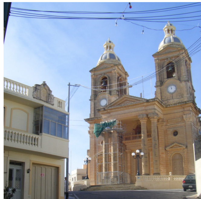
Figure 15.2: View towards the main parish church
