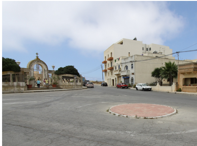
Figure 14.6: Junction A, view of junction towards Triq it-Turretta.
