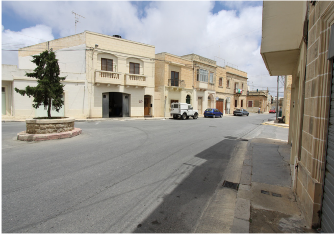
Figure 14.9: Junction B, view towards Dingli centre.
