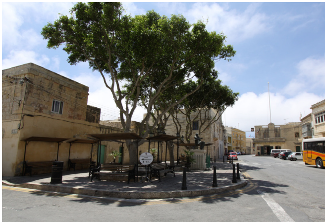
Figure 13.3: The main facade overlooking the open space
