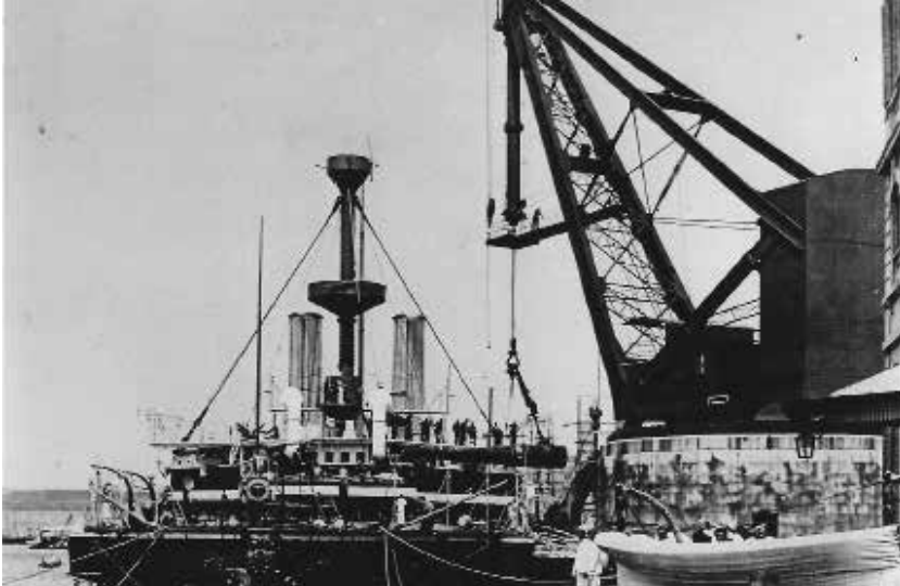
The valve operator on the platform of the 160-ton Armstrong Mitchell Hydraulic Crane hoists out one of the 13.5-inch guns of HMS Trafalgar . Photo published in The Navy and Army Illustrated , 12 June 1896
