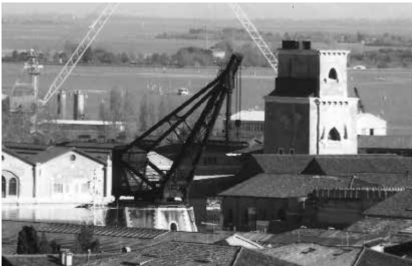
The only surviving Armstrong Mitchell 160-ton Hydraulic Crane is at the Arsenal di Venezia
