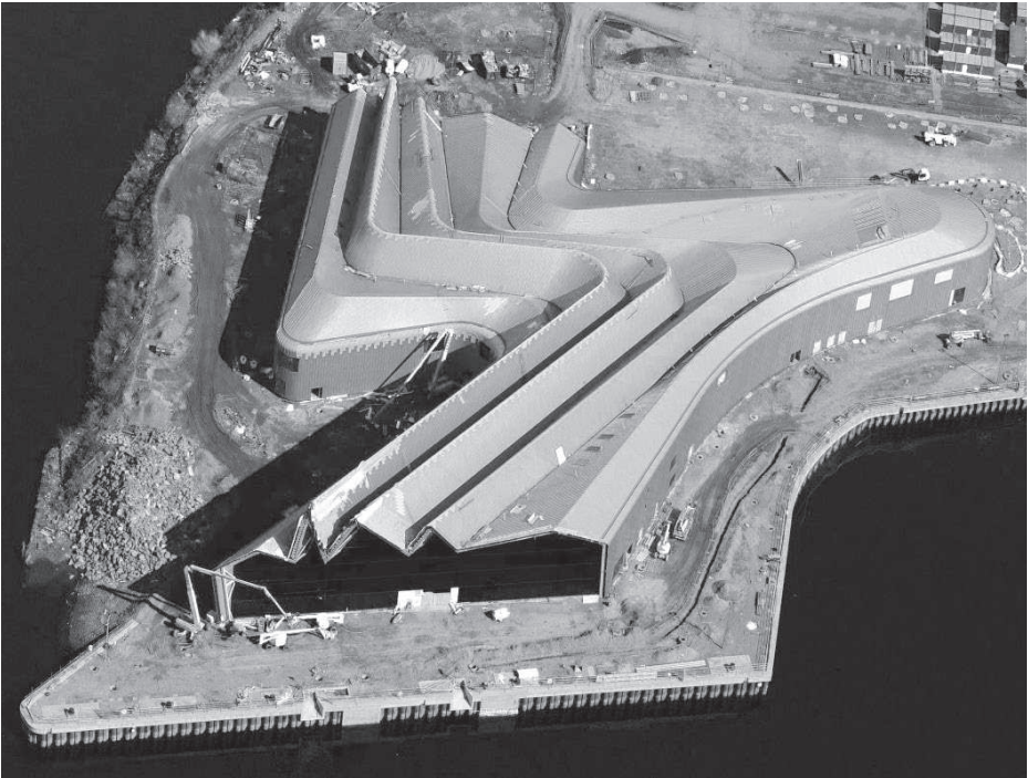
Figure 4. The new Riverside Museum under construction, Glasgow, UK.
