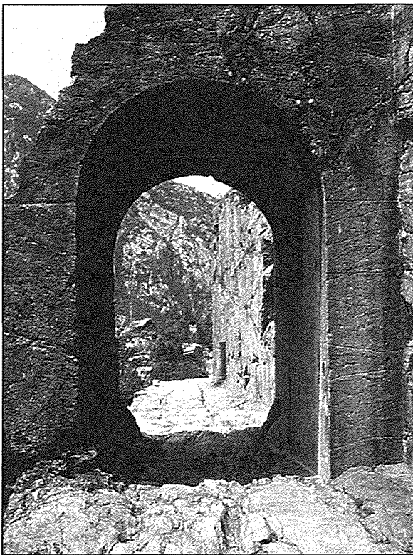
Plate 2: Cart-ruts at Donnaz, Aosta valley, Italy
