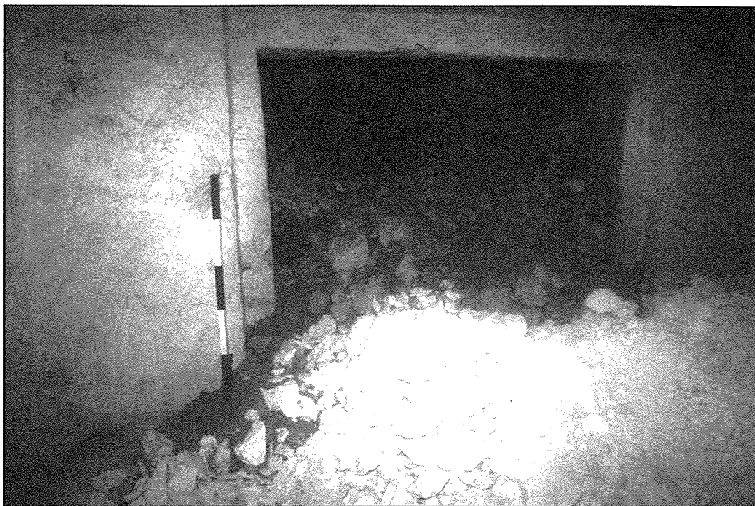
Plate 1: Original entrance containing soil below globigerina chippings
