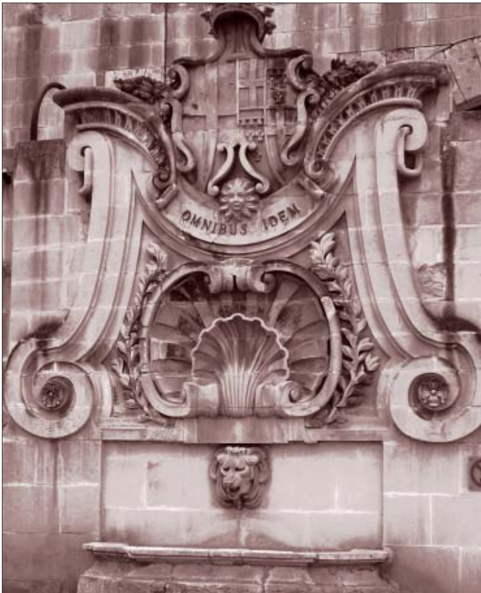
OMNIBUS IDEM (For All Equally): This slogan appears at the top of the first water fountain built in 1615 at the entrance to Valletta, capital city of Malta. The water brought through an aqueduct from the countryside was for the use of everybody equally
