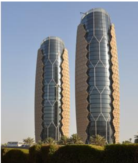
Figure 1: View of the towers from the North
