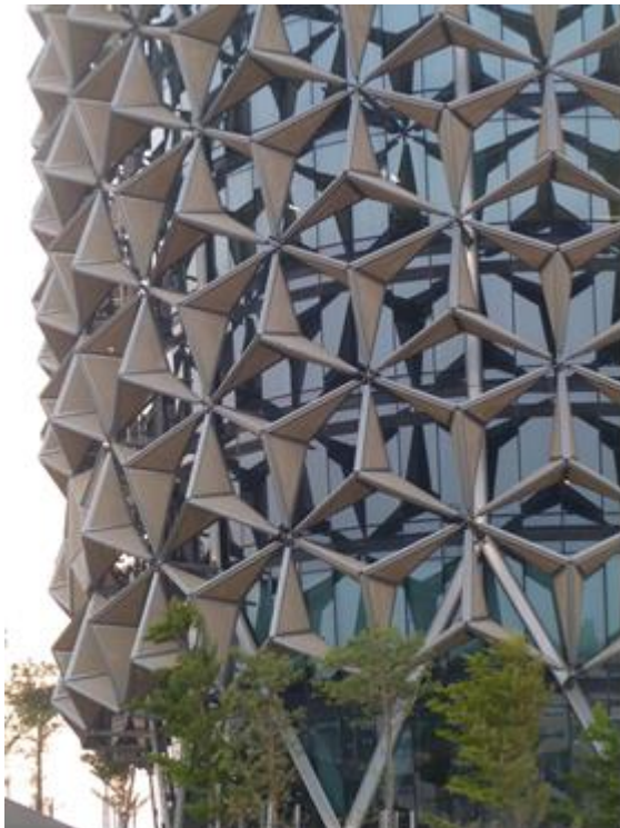
Figure 12: View of lower levels of south east tower
