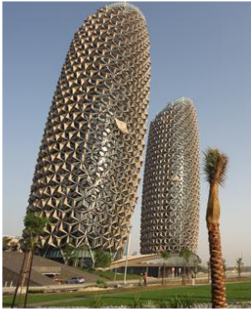
Figure 17: View of completed towers
