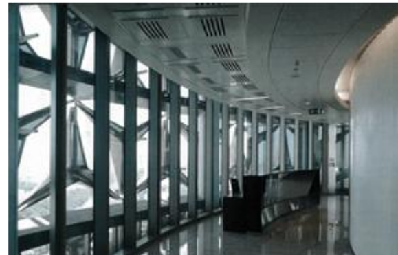
Figure 13: Mashrabiya in open configuration – view from inside office
