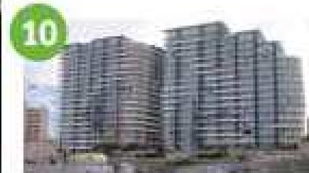
10 SEA-WATER AIR-CONDITIONING SYSTEM AT FORT CAMBRIDGE DEVELOPMENT RESIDENTIAL COMPLEX. Fort Cambridge Development Residential Complex, Tigne, Sliema - Malta
