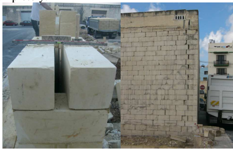
Figure 1: TWO skins of 230mm soft stone with a 50 mm cavity, total 510mm.
