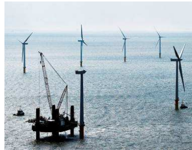
Figure 9: The wind turbine generator being assembled at sea.
