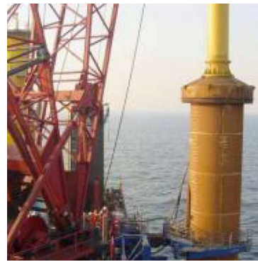
Figure 8: The monopile being hammered into place
