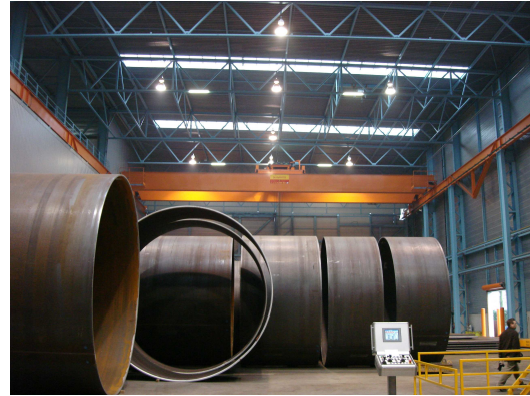
Figure 5: Individual steel cans prior to welding
