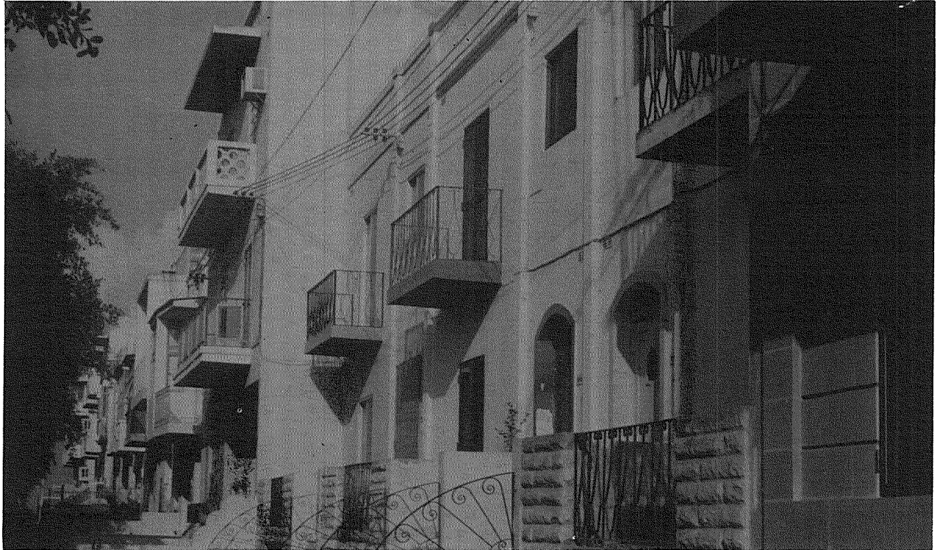
Plate 4: Town houses and apartments built along 21st of September Avenue, Naxxar, during the 1970s had larger balconies and were set back from the road by means of a sidewalk and small gardens or railed terraces.
