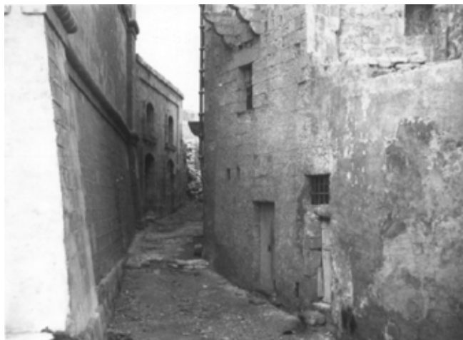
The exponential population increase during the course of the 18 th century necessitated the construction of additional food storage facilities at St Martin's Quarter Street. This 1770s vaulted store currently houses Heritage Malta's Gozo Area Office.
