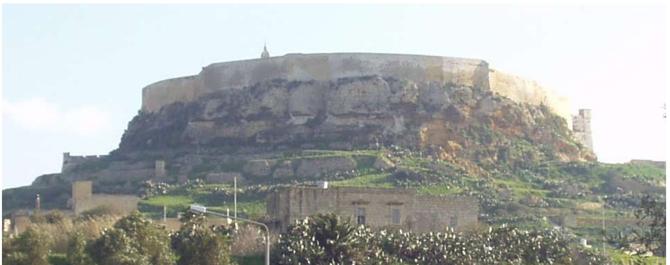
A 2005 view of the north-facing ancient wall of the Gran Castello. Note the then fresh collapse of part of the towering cliff face.
