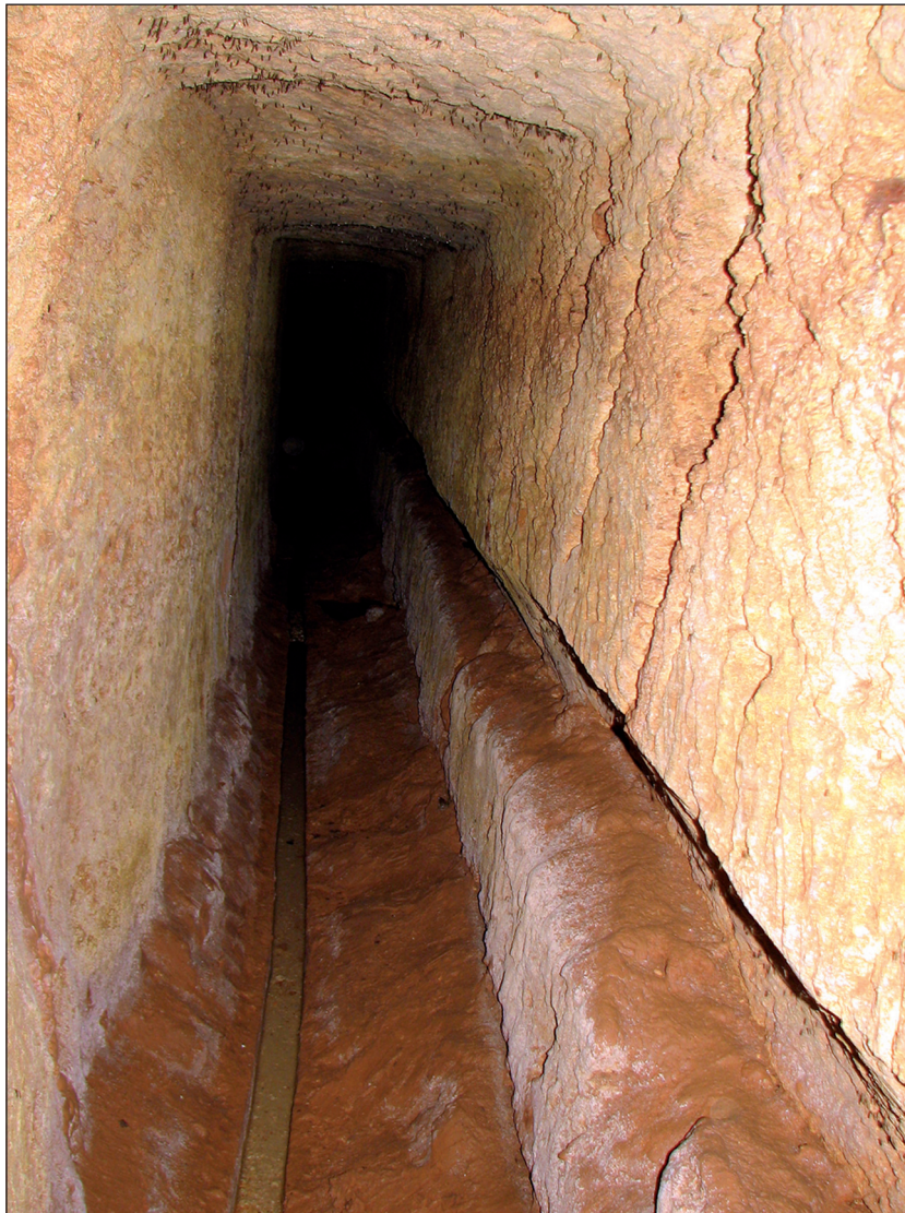
Figure 11.3: Rock-hewn water gallery at Santi, territory of Rabat (Malta). The canal at the base of the gallery channels the extracted water towards the gallery entrance.
