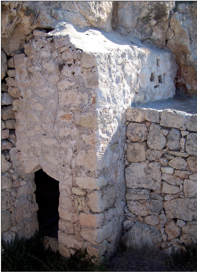
Figure 11.6: Detail of a wet-rubble wall enclosing access to a cave-compound at Bahrija, territory of Rabat (Malta).
