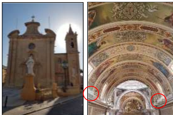
Figure 1: Photographs of the façade and nave with installed AC units of Balzan Parish Church.
