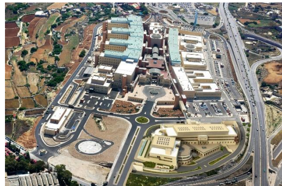
Figure 8: Aerial view of Mater Dei Hospital, Msida
