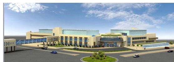
Figure 9: The new Oncology Centre at level 10 with an interconnecting bridge to MDH
