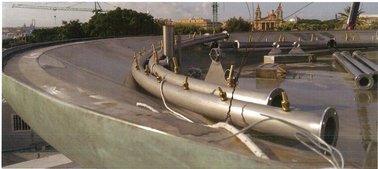
Water nozzles installation in bacino centrale superiore
