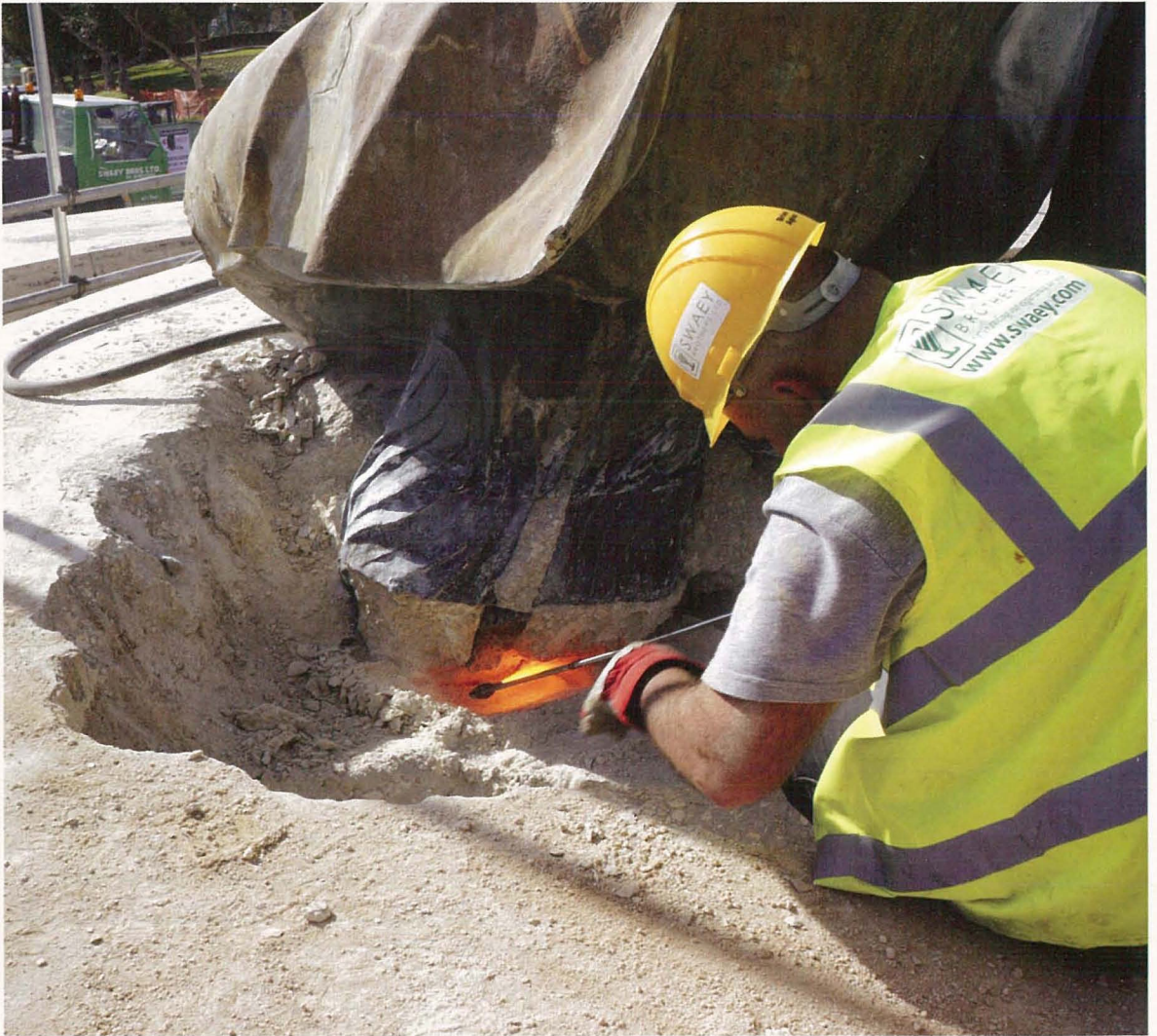
Detaching the steel reinforcement from the concrete screed
