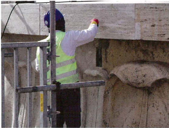
Top left: Micro-sandblasting of vaschetta travertine
