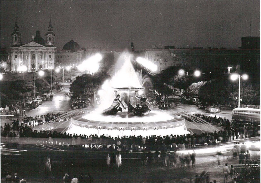
Commissioning of the Triton Fountain on Saturday 16th May, 1959
