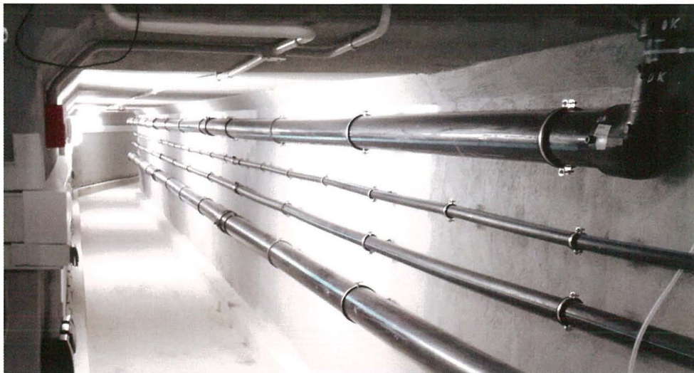
Tunnel connecting plant room to fountain
