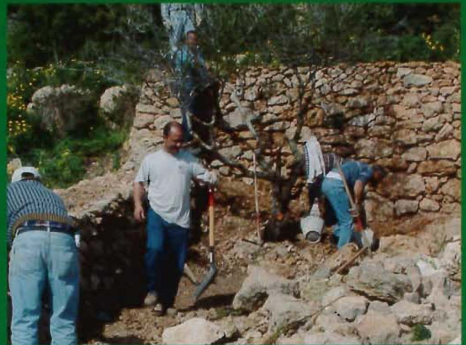
The wall. A team from PARK restoring rubble wall (March)
