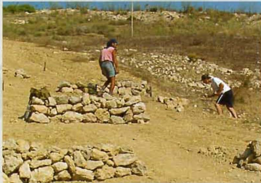
Building barriers. July. Building stone erosion barriers, after their timber predecessors were stolen.
