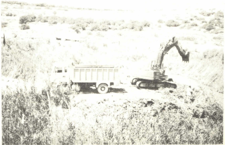
Excavation works being carried out at the Simar nature reserve this summer.
