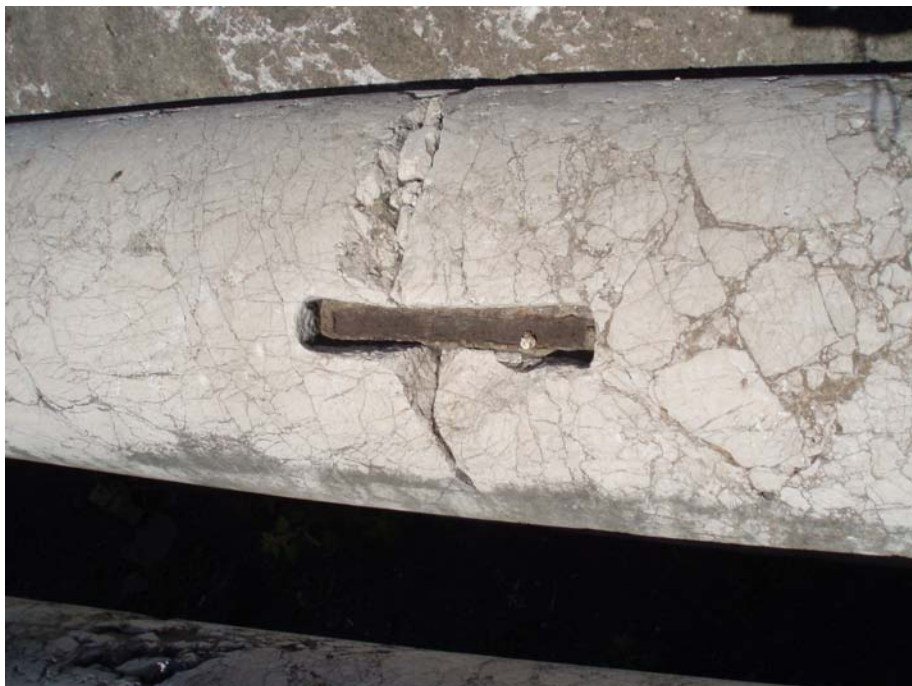
Fig. 14 A repaired column of breccia at the theatre of Catania
