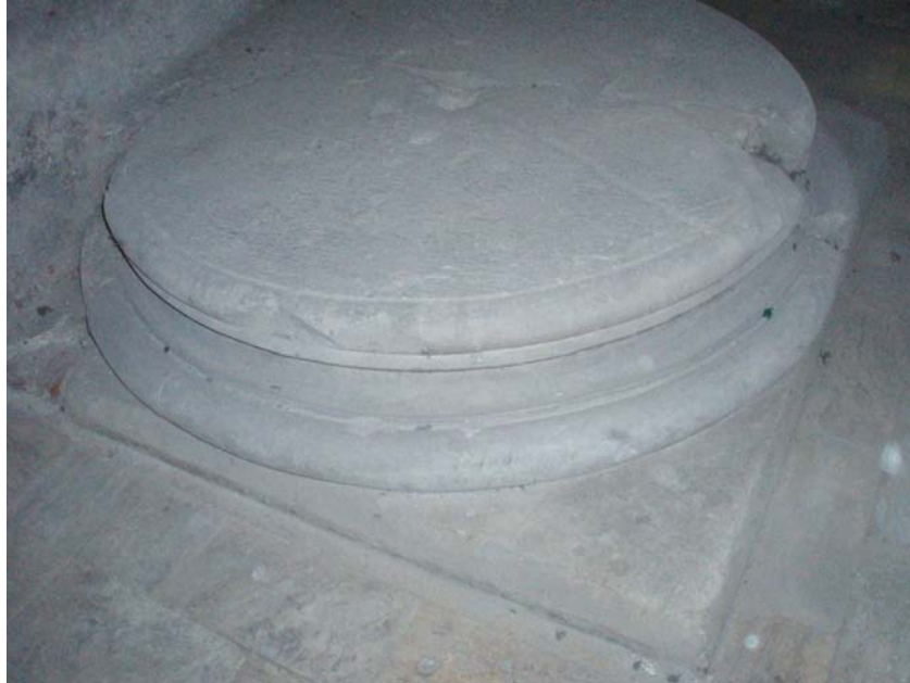
Fig. 28 One of the Byzantine attic bases uncovered in the Cathedral of Catania
