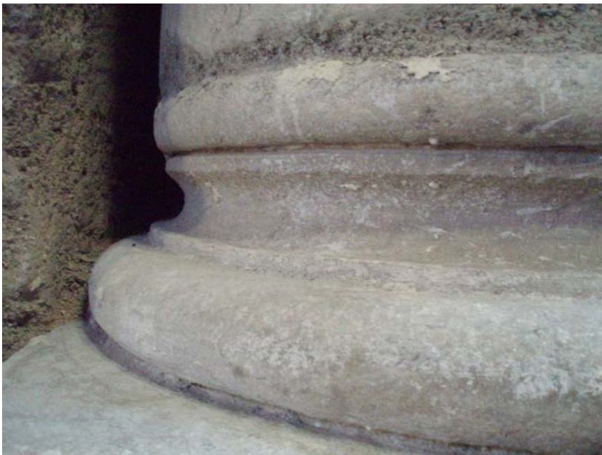
Fig. 24 One of the reused attic bases in the cathedral of Catania
