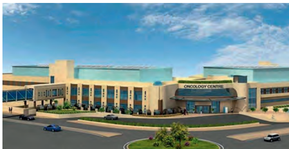
A state-of-the-art oncology centre in Msida
