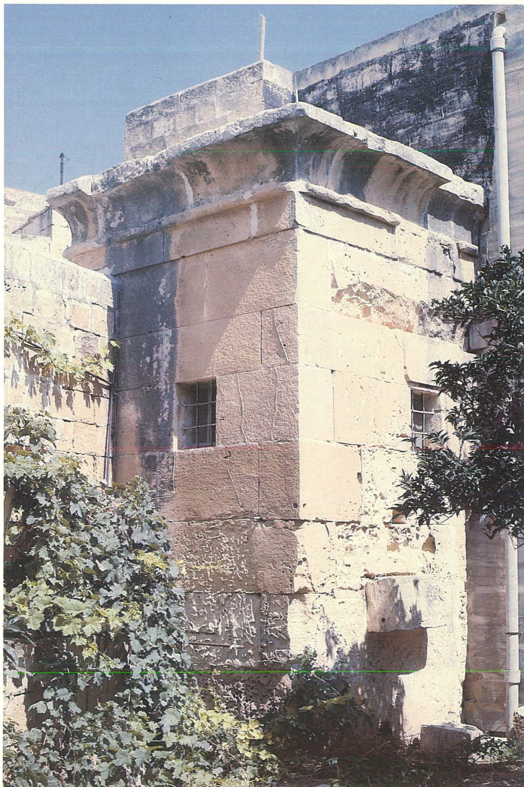
Square tower (5.60m. high) of ashlar masonry, datable to the late Punic period, inside a private garden in Żurrieq.
