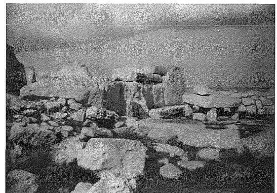
Plate 5. Façade of the main building at Haġar Qim after repair of the lintel and restoration of upper courses in 1910. (National Museum of Archaeology)
