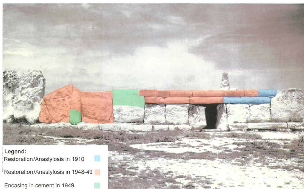
Plate 9. Different phases of restoration of the façade of Haġar Qim
