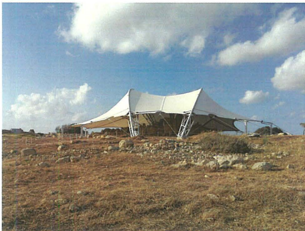
Figure 1. Hagar Qim and its protective shelter (photograph by Simon Farrugia).
