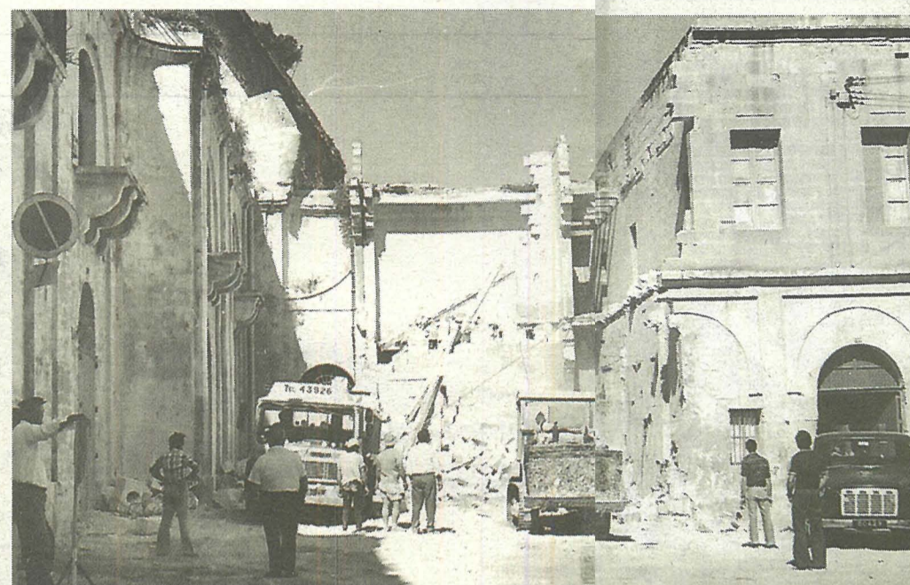
1978: Demolition work revealed part of the former Consegna...
