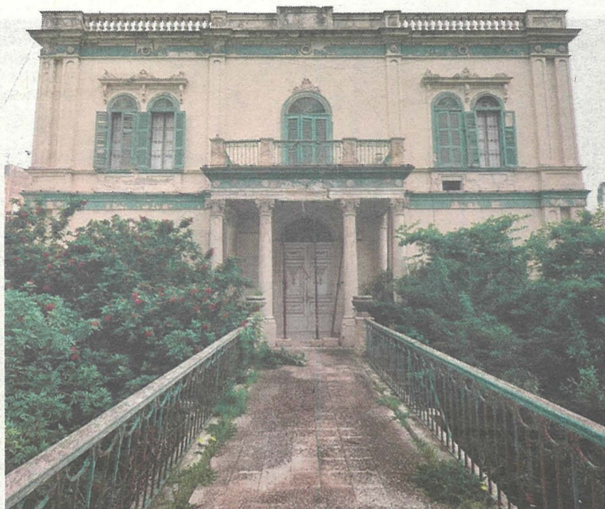
Before: View of current Villa Drago facade.
